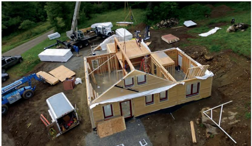
After your building shell is up, the post-assembly work can be completed, including the electrical, plumbing and HVAC work, and exterior and interior finishes. While many factors affect the project schedule, a Unity Home can be completed as quickly as 6-10 weeks after the weathertight shell has been assembled on site.
