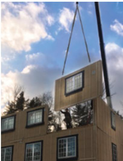
**SHELL** Unity assembles the high performance building shell of your home on site (wall, roof and floor components along with windows, doors and interior partitions.) We coordinate with the local builder who installs the foundation, and finishes the exterior and interior of the shell we erect.
